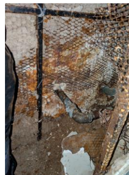
Missing insulation on cold water supply t
