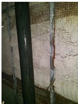
Missing insulation on cold water riser
