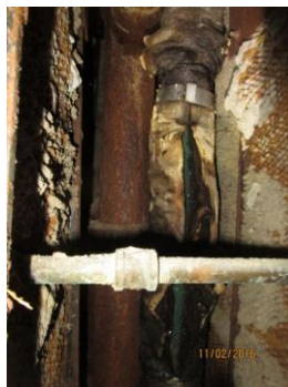
Damaged insulation on cold water riser
